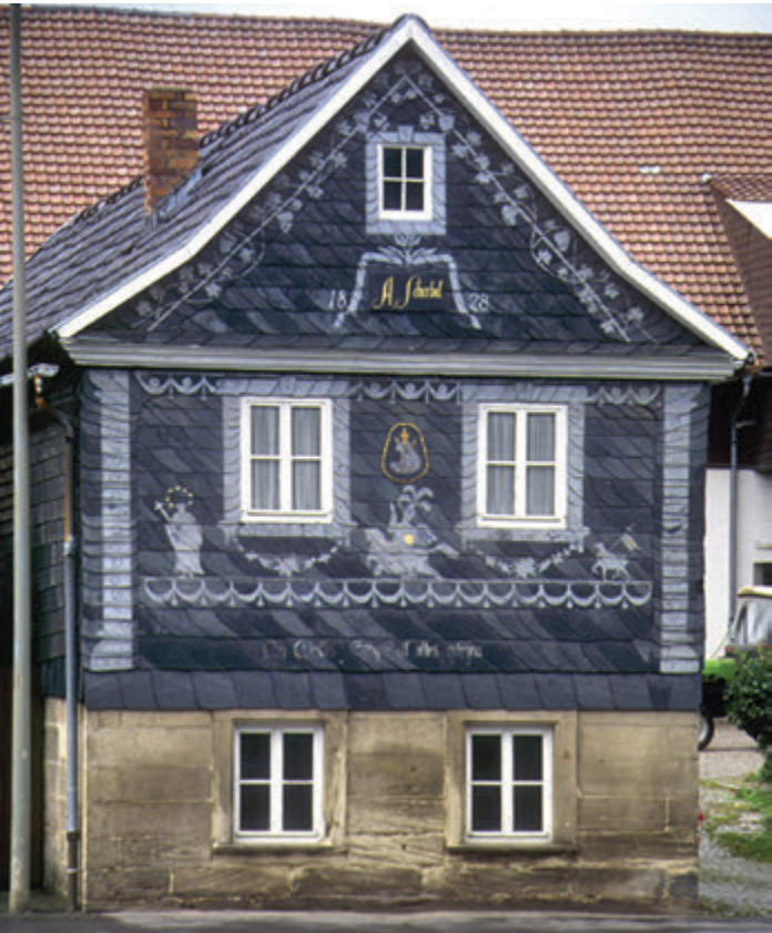
Slate façade from 1828 with later renewed decorations with tin foil ('Stanniol'), typical of northeastern Bavaria. Photo: S. Scheidig
