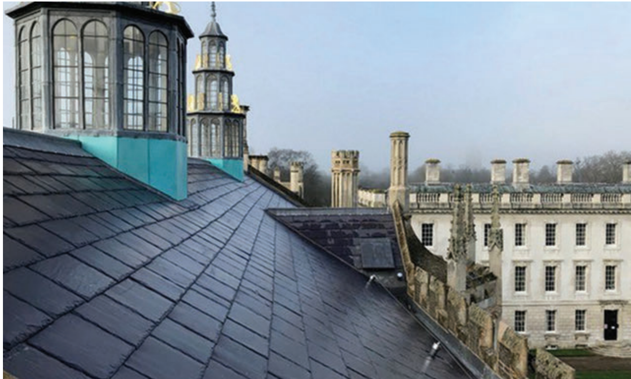
Typical roofing with Welsh slate
