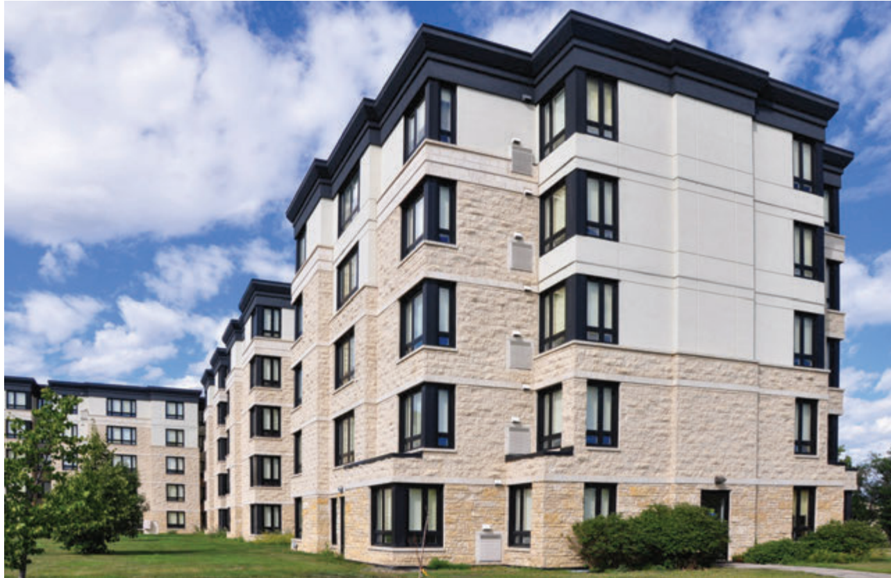
Student residence, University of Saskatchewan, Saskatoon. The first floor has rustic finish from slabs split along bedding plane-parallel stylolites. Second to fourth floors are split-face blocks. Decorative courses are sawn parallel to bedding.
