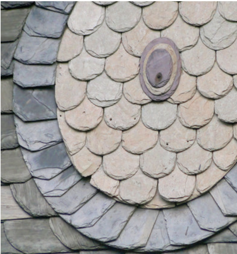
Slate wall cladding with the previously existing 3 slate colours (from outside to inside: black, green, purple) (figure diameter approx. 2.5 m) (over 100 years old).
