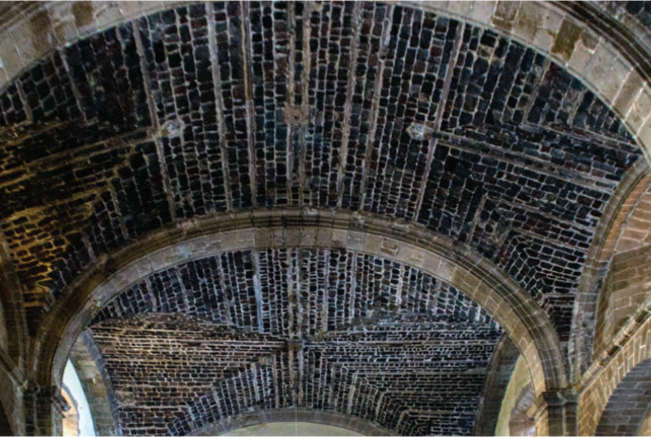
Choir vault built with tezontle to achieve a weight-reducing effect- a constructive innovation of the 17th century in Novo-Hispanic architecture-. The ornaments on the cusp are carved in clear tuff. Example from the Baroque-style San Lorenzo Mártir temple, Mexico City.
